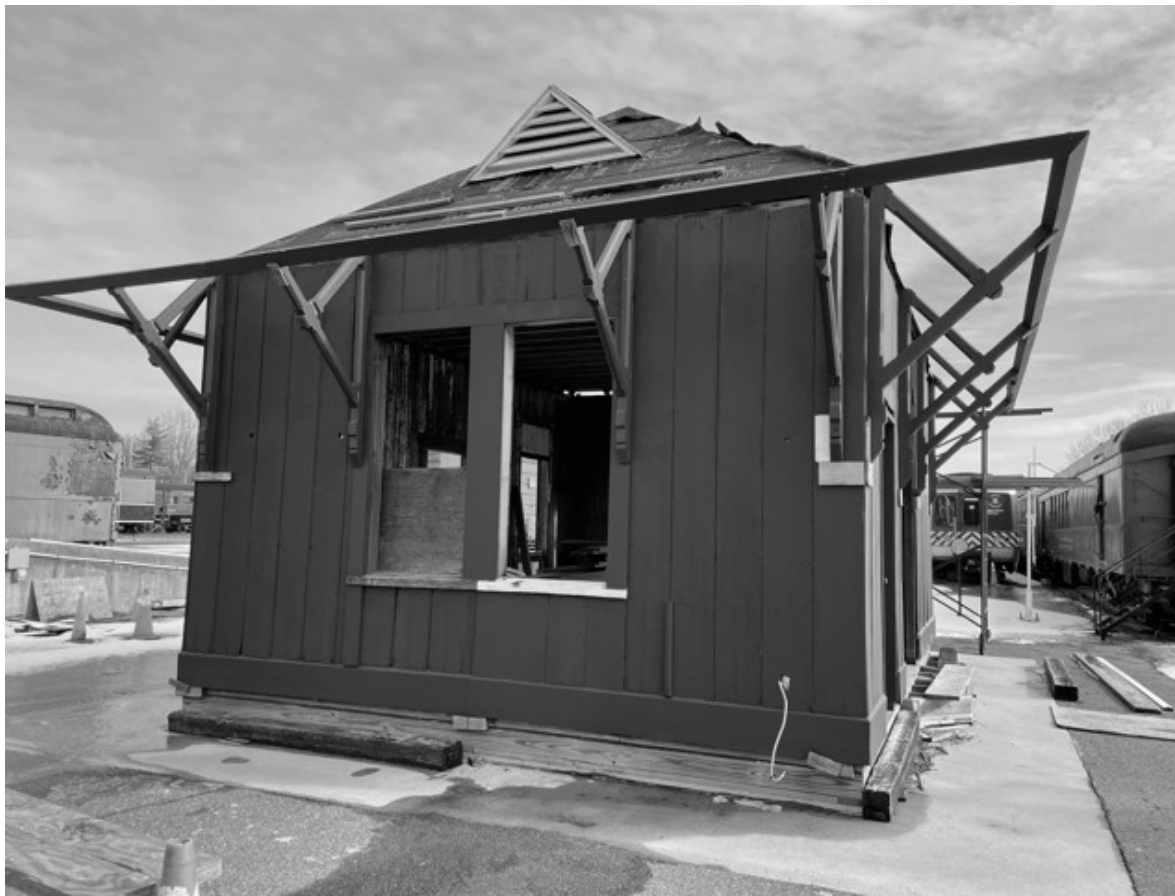
ROOF FRAMING WORK DONE AND SIDING REPLACED – Progress being made.
