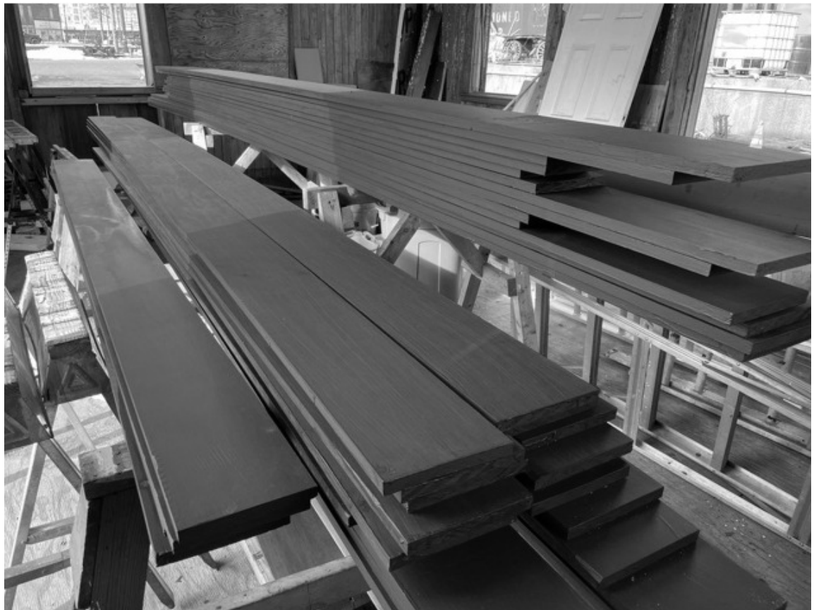
CANOPY RAFTERS, BRACKETS RECONSTRUCTED – Volunteers scraped, painted to match originals.
