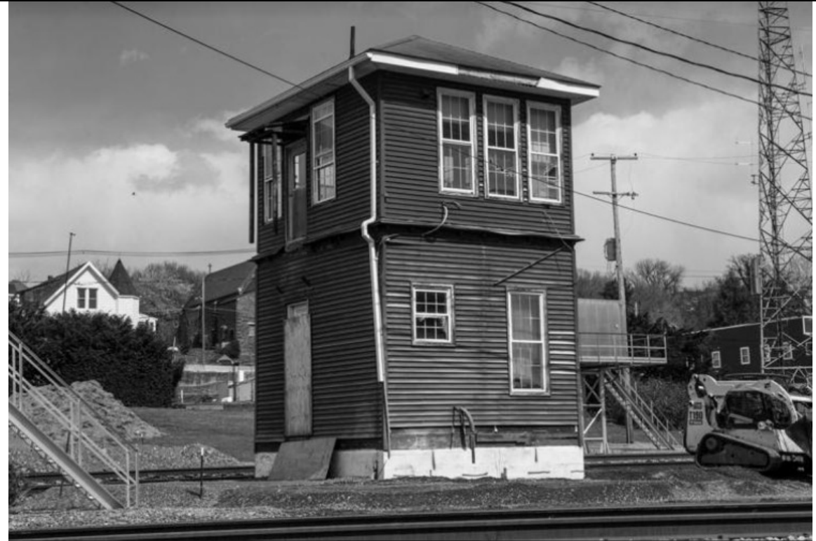
WEST BRUNSWICK TOWER IS THE LAST-REMAINING HISTORIC STRUCTURE ON THE 93.5-ACRE RAILYARD OWNED BY CSX TRANSPORTATION – Built in 1910 by the Baltimore & Ohio Railroad, the building was taken out of service in 2011 by CSX.
