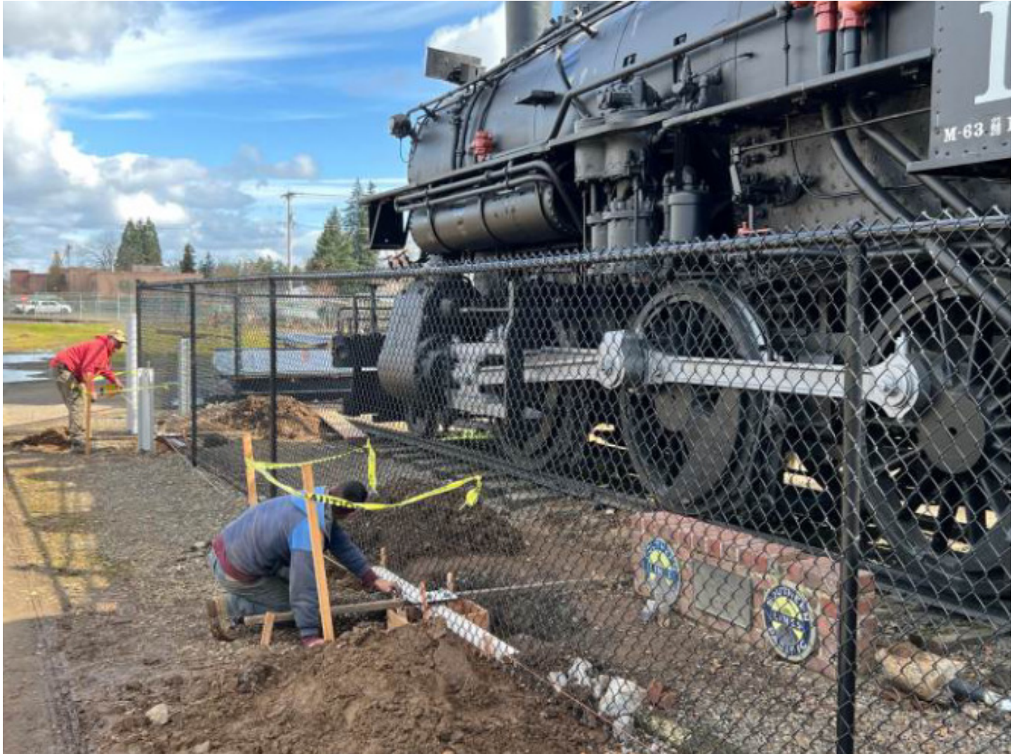
CONTRACTOR WORKS ON MARCH 16, 2022.
