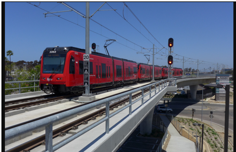
INBOUND TRAIN ON BLUE LINE EXTENSION MUCH OF WHICH IS ON AN ELEVATED STRUCTURE.
