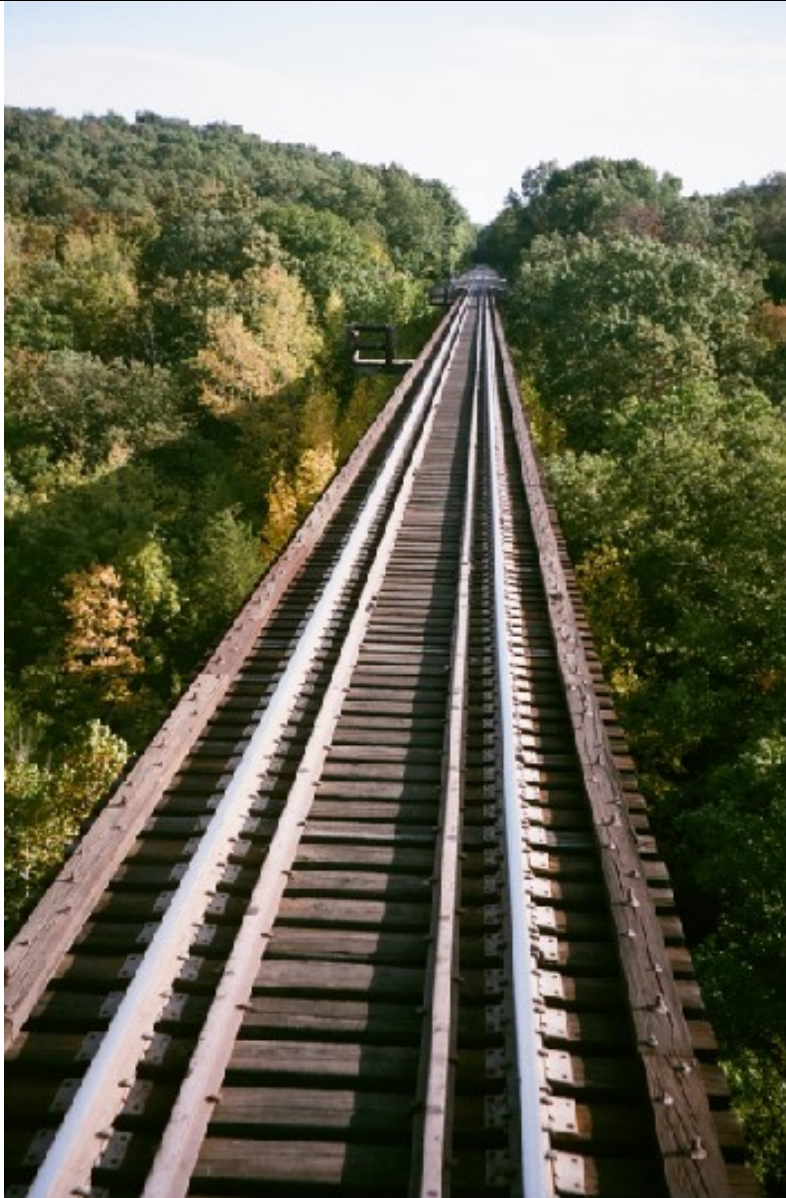
PHOTOS COURTESY OF ELIZABETH GUENZLER VIEW FROM THE REAR PLATFORM OF A&M "EXPLORER". This is the second of three trestle bridges on the Arkansas and Missouri line to Van Buren, Trestle Two stands 110 feet high, is 431 feet long and is known as the Boston Mountain Viaduct 2.
