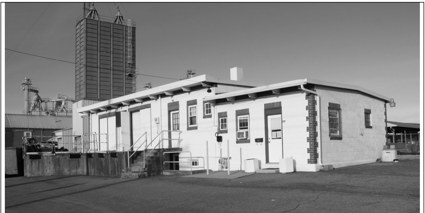
FORMER PENNSYLVANIA / PENN CENTRAL FREIGHT STATION ON DECEMBER 10, 2022 – For 75 years, the freight station at New Holland Pennsylvania served as a centerpiece among several rail sidings in the vicinity of MP 28 of the current Norfolk Southern New Holland Secondary.
