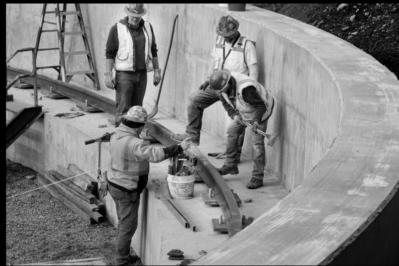
FINISHING THE CENTER PIVOT – To be used for the bridge.
