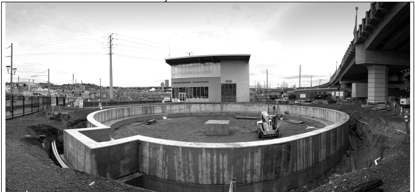
FINISHED CONCRETE STRUCTURE – To be used for mounting the turntable bridge.
