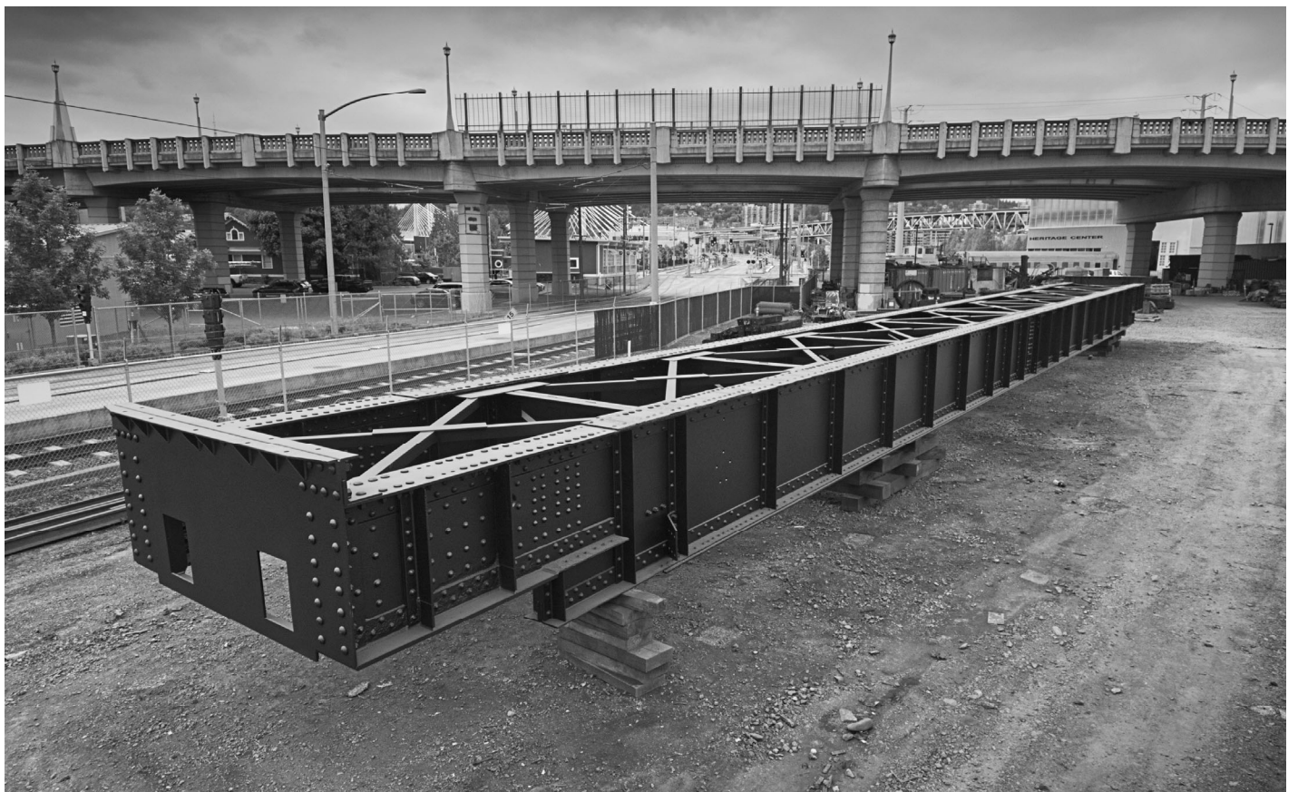
THE RESTORED BRIDGE – This turns the locomotives.
