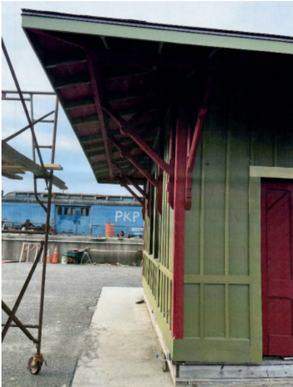
DETAILING COMPLETED ON SIDES AND ON ROOF - Frieze boards, corner boards and battens are installed.
