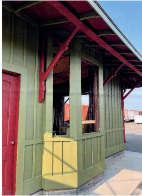
AGENT'S BAY REPAIRED - Sills, window have been installed for the agent's window as well as siding and battens.
