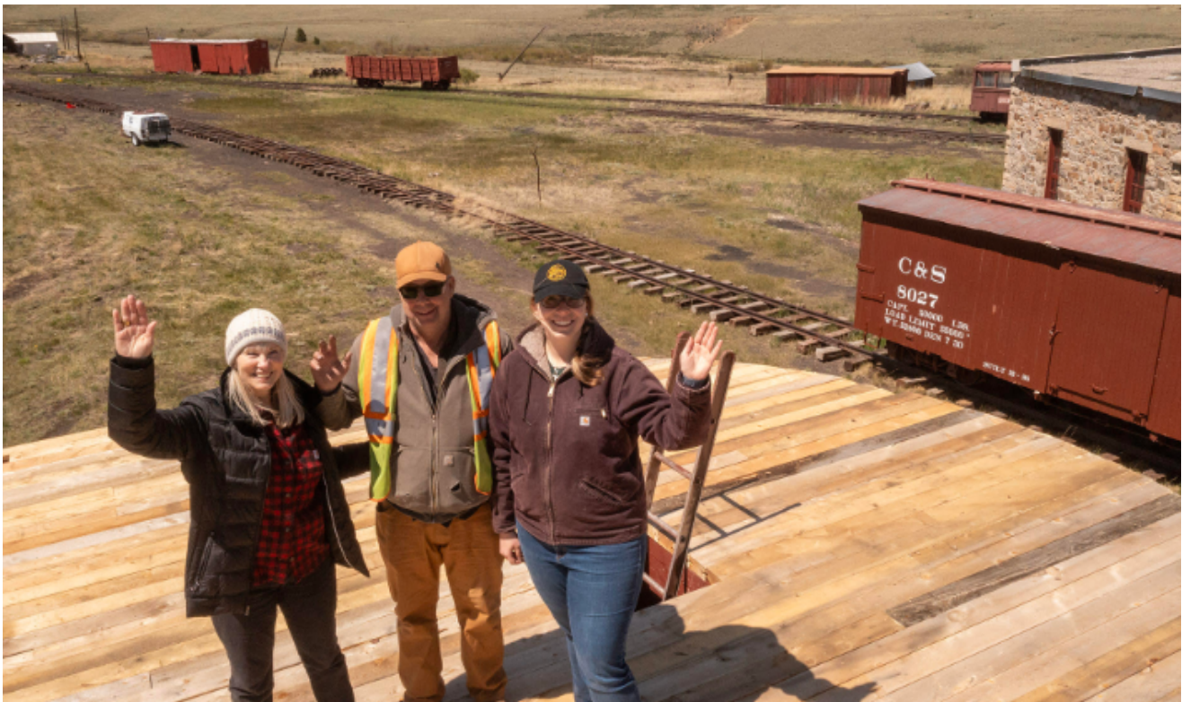
DENVER, SOUTH PARK & PACIFIC HISTORY SOCIETY WATER TANK IN COMO, COLORADO - Left to right, Kathy Brantigan, Bob Revis, and Lauren Revis on upper platform of newly constructed water tank.
