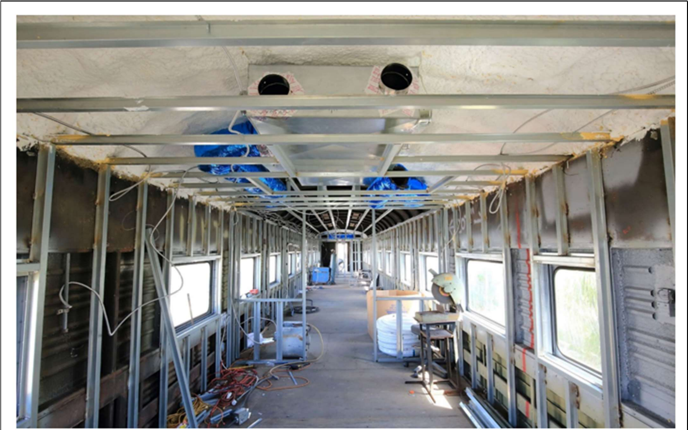
INTERIOR UPDATE 1 – Included HVAC and electrical work.
