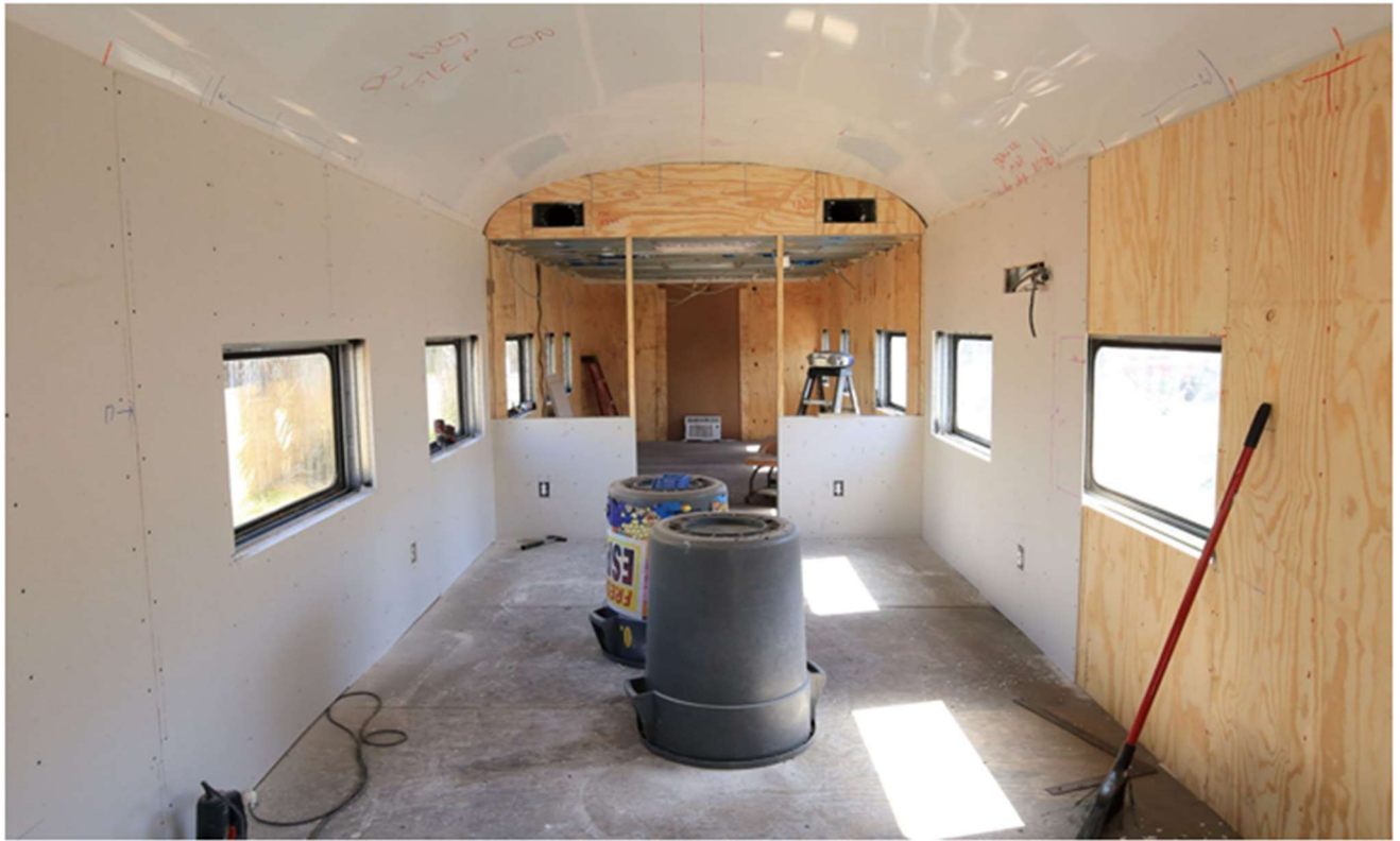
INTERIOR UPDATE 3 – Finishing the clean-up before adding interior rooms.
