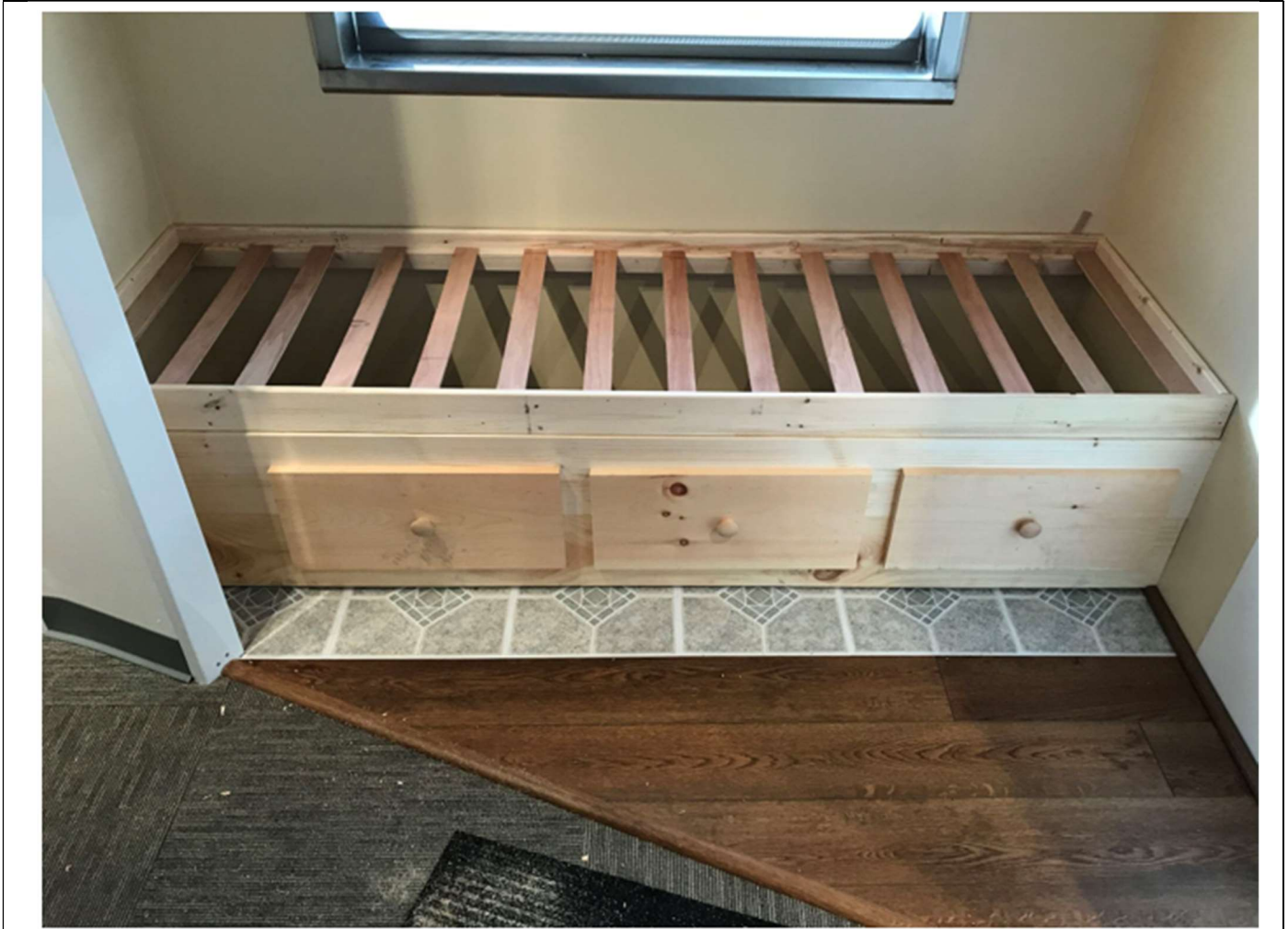
INTERIOR WORK – Finishing the details.
