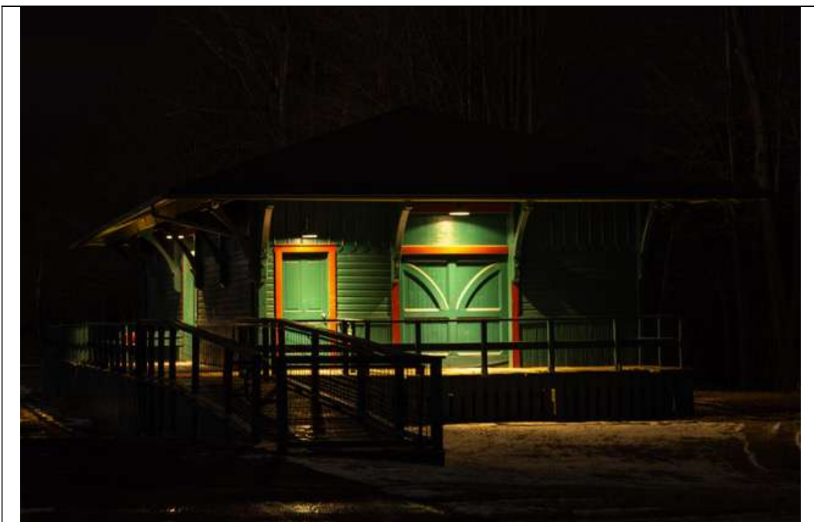
MOSCOW FREIGHT STATION – Appropriate for a Freight Station, the new lights are powder coated in a dark green that goes with the station colors.
