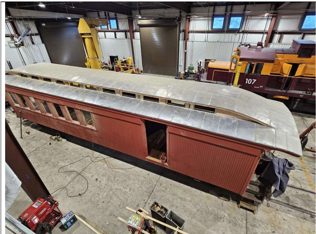
WORK UNDERWAY – As of January 2025.
