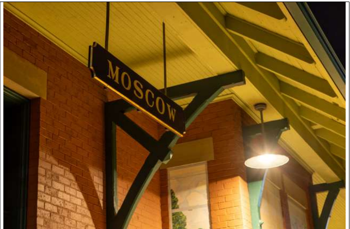
MOSCOW STATION – New period light fixtures suitable for the age of the station.
