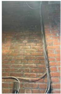
Above: Damage to walls in the tower's first floor, southeast end, near the diorama area, showing how water seepage has discolored the bricks.
