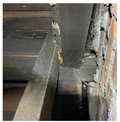
The main beam is cracked at the lower section due to stress from water, fatigue of the rafters, and weight, probably due to snow buildup. It is sagging by about 2 inches and will need to be bolstered to restore its structural integrity.
