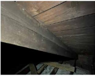
This attic view shows the stress in a rafter, the only one that's damaged so far. It's in the southeast corner, where most water is entering the property.
