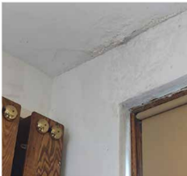
Water damage in a corner of the attic. The dark coloration of the brick shows where water has been penetrating from the roof line.
