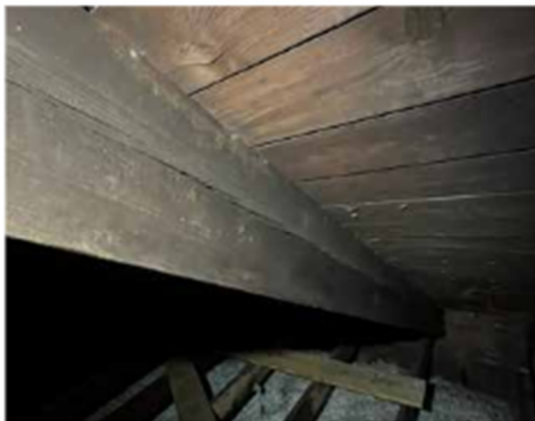
This attic view shows the stress in a rafter, the only one that's damaged so far. It's in the southeast corner, where most water is entering the property.
