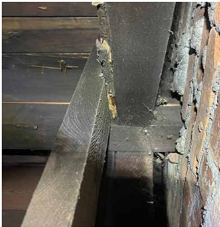
The main beam is cracked at the lower section due to stress from water, fatigue of the rafters, and weight, probably due to snow buildup. It is sagging by about 2 inches and will need to be bolstered to restore its structural integrity.
