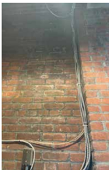
Above: Damage to walls in the tower's first floor, southeast end, near the diorama area, showing how water seepage has discolored the bricks.
