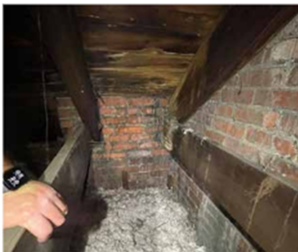
Water damage in a corner of the attic. The dark coloration of the brick shows where water has been penetrating from the roof line.
