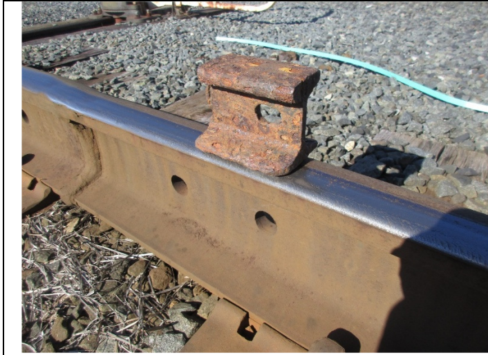
FIGURE 1 - Section of an original Camden & Amboy Railroad flat-bottom T-rail on top of a modern flat-bottom T-rail.
