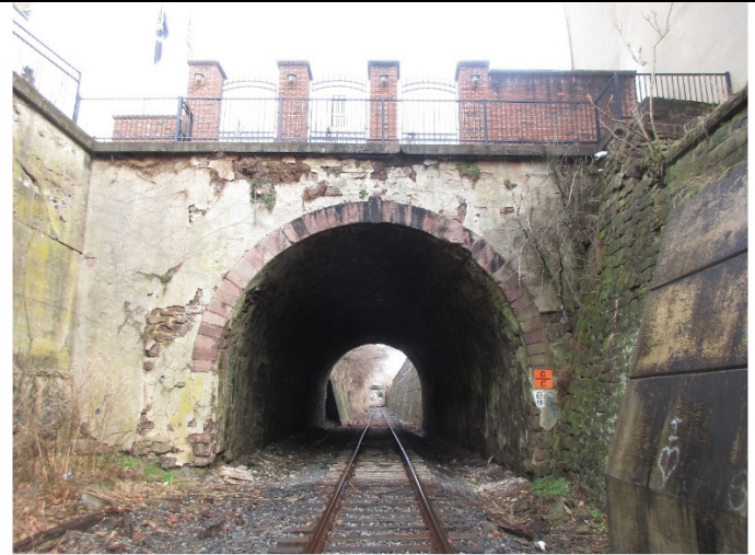
FIGURE 2 - West entrance of the Camden & Amboy Railroad Farnsworth Ave. Stone Arch Bridge built in 1831. The oldest active bridge built over flat bottom T-rails in the world.
