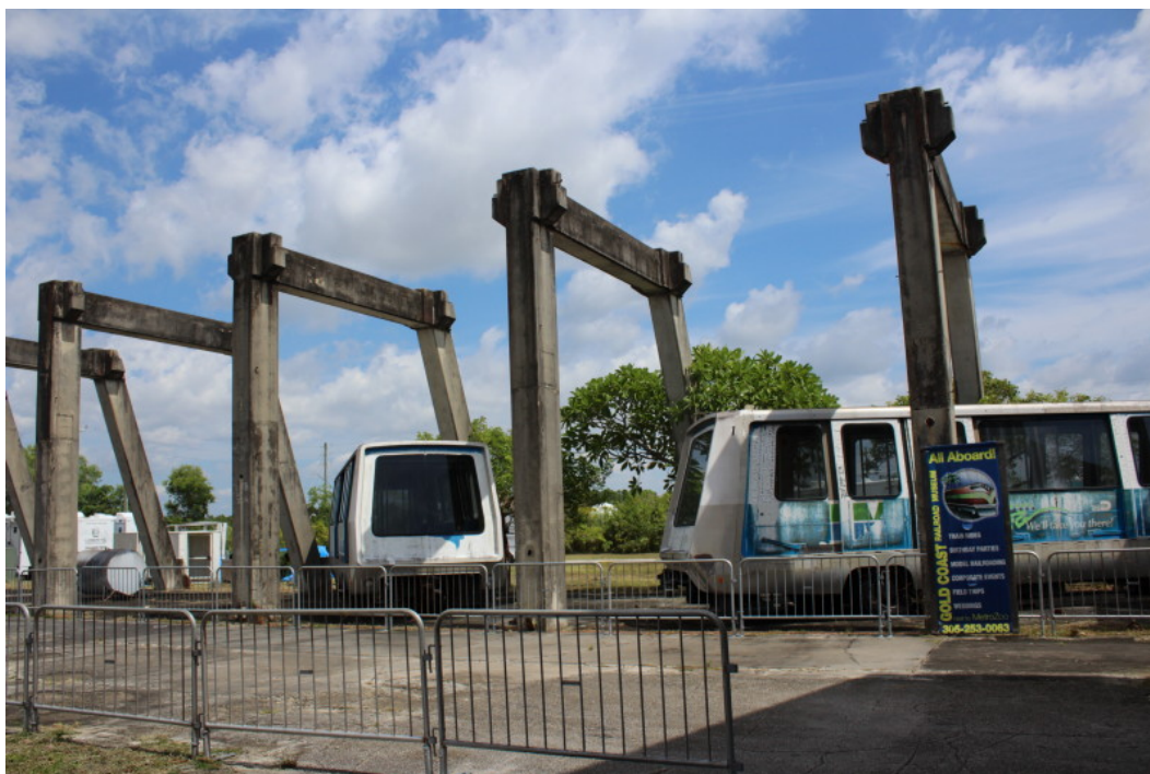
The Gold Coast Railroad Museum is housed at the former Richmond Naval Air Station, a "lighter-than-air" blimp base that operated between 1942 and 1945. Three years to the day after decommissioning, the base was destroyed in a hurricane and fire. The vehicles are the original Miami Peoplemover on display with the remaining concrete supports for the fifty-one wooden truss arches of hangar 1. Photo by Robin Bowers.
