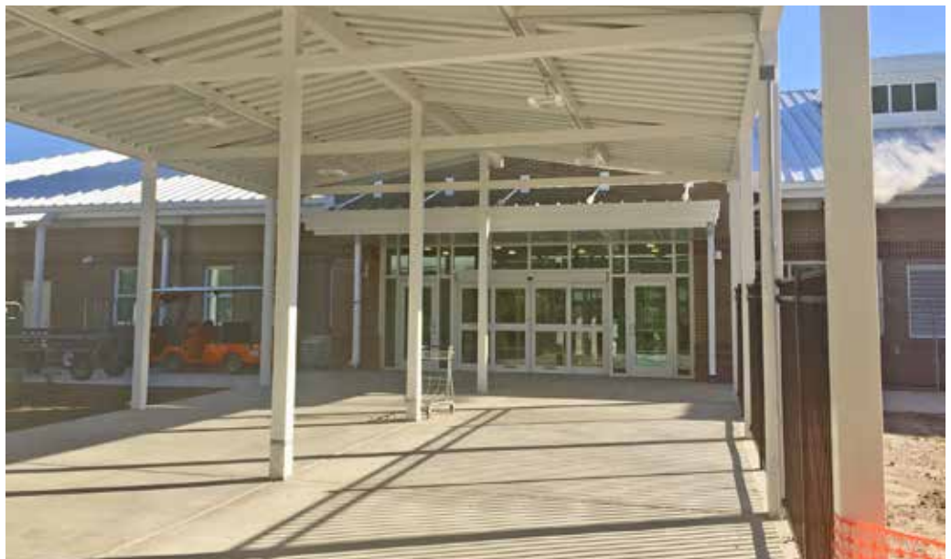
SHOWN IS THE TRACKSIDE ENTRANCE to the new depot in Charleston.
