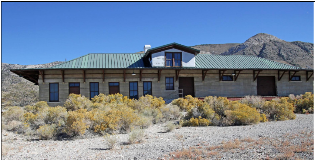
NEVADA NORTHERN LINES TOWARDS COBRE, NEVADA - This is the historic passenger depot in McGill, 16 miles north of Ely, built in the early 1900s. The railroad already owns the McGill depot and has spent hundreds of thousands of dollars restoring it to its former glory. The Nevada Northern Railway Museum has recently been awarded a $10 million grant to rebuild 16 miles of railroad from Ely to McGill and install a turntable here.
