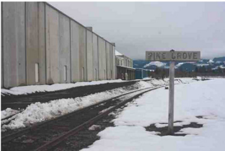
Buildings at Pine Grove (Photo by T. Trent Stetz)
