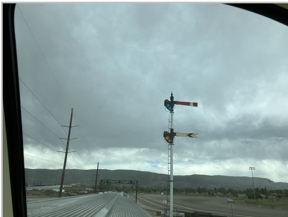
A double lower quadrant semaphore signal as seen from the dome car, just beyond the yard.
