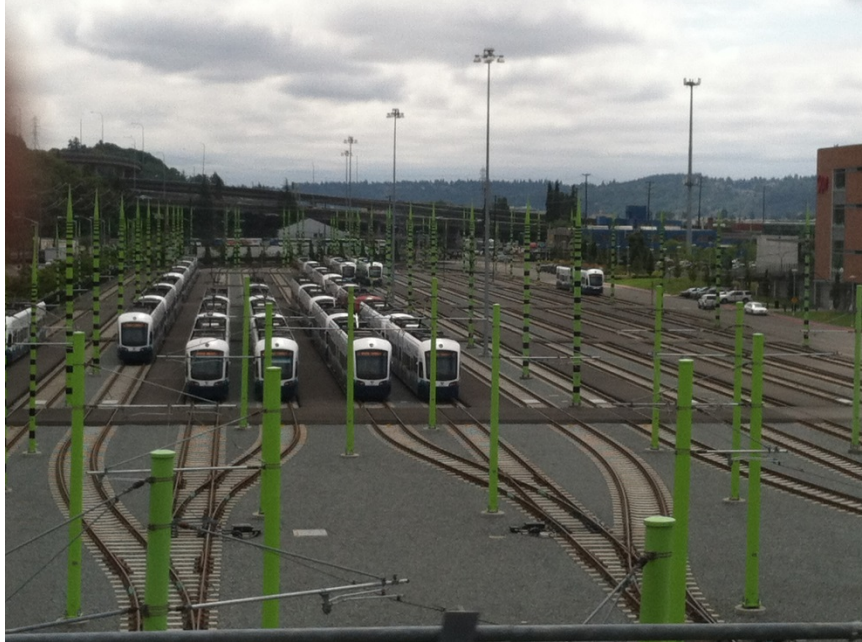
Seattle Central Link – Operations Maintenance Facility
